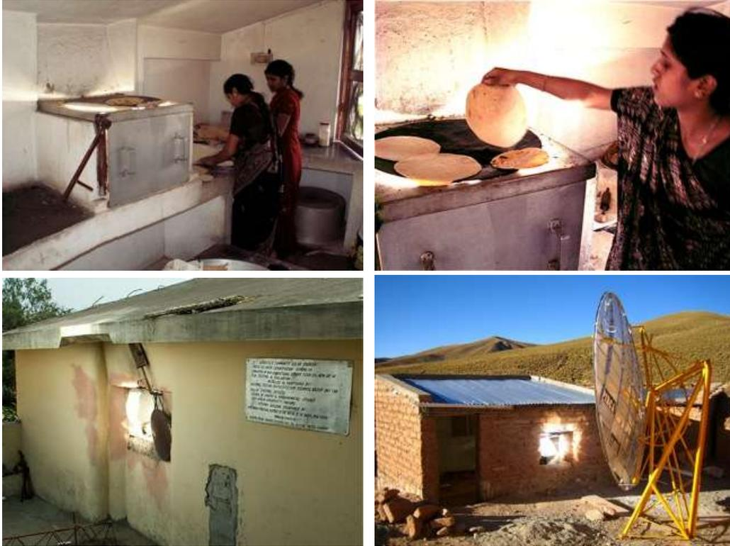
One of the Scheffler reflectors at Barli Institute [heats a storage unit](#), which allows cooking at night.
