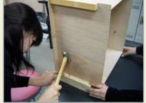
7. The outside boards (Boards 7, 8, 9, and 10) should now be fixed to the pillars (B) which are attached to the inside boards. Use both the PVA wood glue and 25 mm nails to fix the outside boards one at a time to the pillars (B). Pack insulation tightly between the inside wall of the box and the outside wall of the box.
