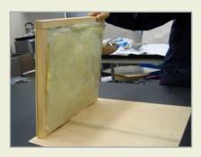
5. Take the inside boards (Boards 3, 4, 5, and 6) one at a time and place them vertically and in line with the edge of the inside bottom board (Box 1). Where one of the vertical edges should align with adjacent side of the inside bottom board for the inside box (Box 1) and the other end 4 mm from the edge of the bottom board for the outside box (Box 2). Using PVA wood glue and 25 mm nails, fix the four inside boards to the frame separating the bottom boards.
