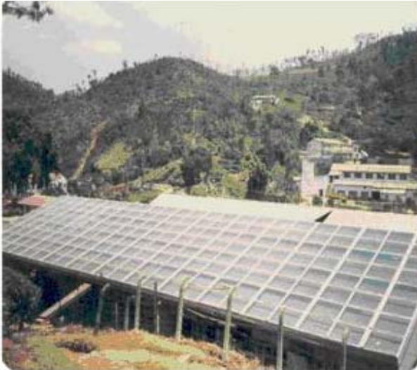
Golden Hills 212 m 2 Installed In 1992
