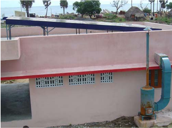
SOLAR FISH PROCESSIN PLANT AT POOMBUHAR, TAMILNADU
