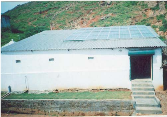
SOLDRY- FISH PROCESSING FACILITY PLANT, AT DFYWA, VISAKHAPATNAM
