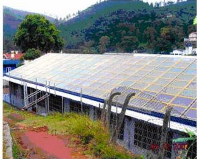
Unit after 15 years with repainting – 2007 December
